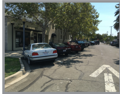
Angled Parking on 3rd Avenue
