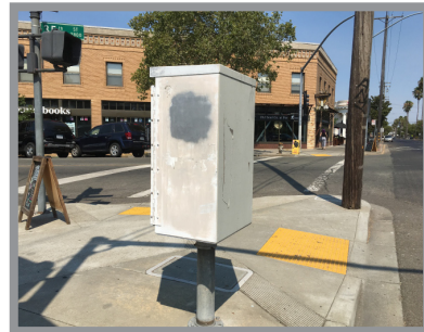
Utility Box at 35th/Broadway
